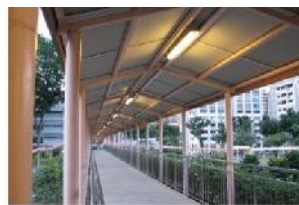
Pedestrian overhead bridge
